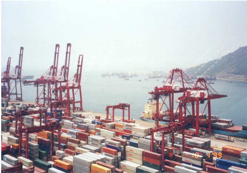
Fig. 1. The container storage yard in a terminal with containers stored in columns or stacks of four to six containers. RTGCs (Rubber Tyred Gantry Cranes), which help to stack containers and retrieve them, can also be seen among the containers. The storage yard is divided into rectangular areas called blocks.
