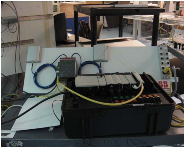
Figure3: Test setup with the I/O module
